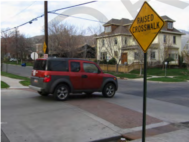
This raised crosswalk on 2nd Ave calms speeds and elevates the crossing for better visibility
