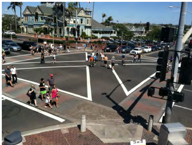
Scramble in Carlsbad (CA) that serves 8,000 pedestrians per day
