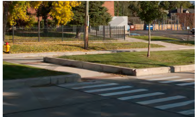
Median refuge island near Bennion Elementary on 800 East
