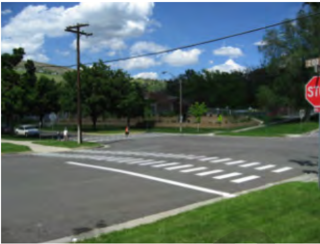
Salt Lake City uses double ladder crosswalks in school zones and at midblock crosswalks in the downtown Central Business District
