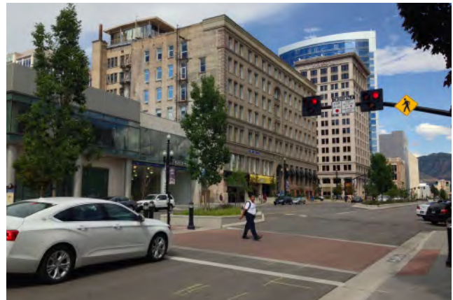
HAWK signal on 100 S between West Temple and Main St
