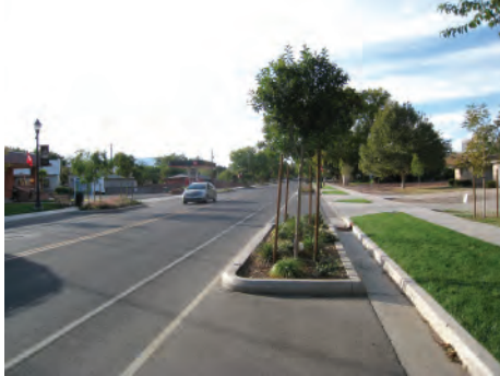
Planters and curb extensions in the parking lane on Sunset Blvd in Santa Clara, UT
