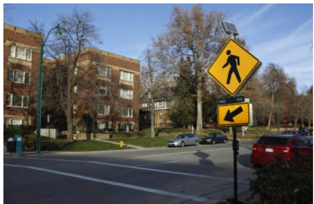
RRFB pedestrian crossing at 1100 East South Temple
