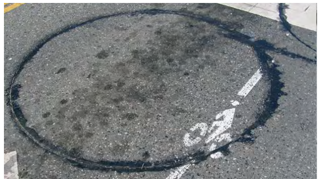
Standard loop detection pavement marking (Photo: NACTO)
